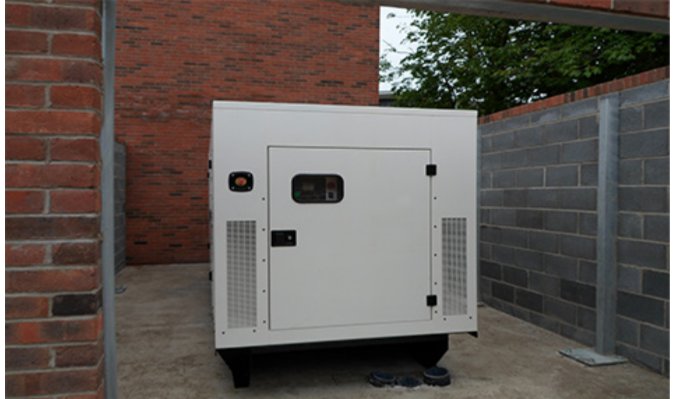
500kVA Diesel Generator Installation
